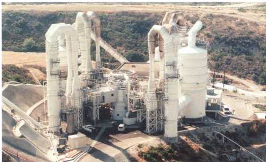
The California site of the TRW Strategic Defense Initiative (SDI) laser project is one of the world's largest vacuum and air pollution control installations. Ejectors manufactured by Croll-Reynolds simulate the atmosphere of space for the testing of a hydrogen/fluorine laser. Gases produced during laser generation are removed by a Croll-Reynolds custom-designed Packed Tower Scrubber.
