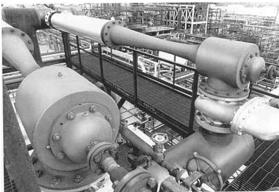
In the Petrochemical and Chemical Process Industries, Croll-Reynolds' Thermocompressors recycle waste steam and reduce energy consumption by 30% or more.
