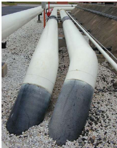
Main hydrant pipes disappearing into the ground
