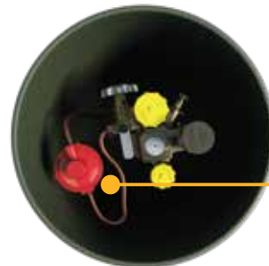
Installed above highest probable water level
