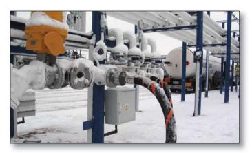
The TODO® SAFETY BREAK AWAY coupling are designed to eliminate spillage and damage associated with drive / pull away incidents. Offer exceptionally high flow capacity for their size.
