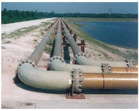
Ninety degree sweep elbows lined with ceramic tiles are one of the fittings choices you have when designing a complete CERAM CORE piping system.
