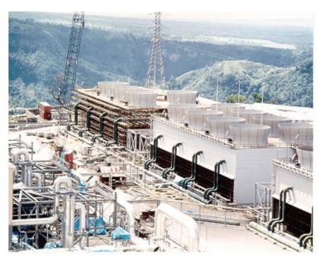
F-CHEM custom piping is supplied for condensed steam cooling tower supply and return lines at geothermal power plant.
