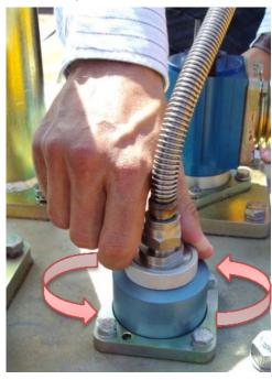
3. Part way through a normal tanker delivery (when tank is above 80% full), depress the test top of the sensor cartridge.
