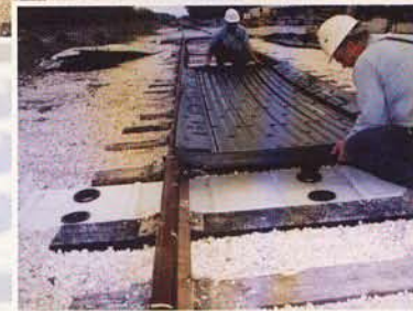
EXTEND BALLAST SHOULDERS BOTH SIDES OF TRACK OUT FROM RAIL A MINIMUM OF 4'-0" WITH LIMITS OF ENVIROPAN INSTALLATION
