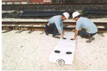
5. In tangent track, make sure that the cross drains are placed in the track 90° to the rail. This can be done by marking desired center of cross drain on rail. Measure 36' down rail from mark. Measure 67" from mark diagonally to opposite rail. The two marks on the rail must be lined up with center of cross drain. Contact Century if the track is not tangent.
