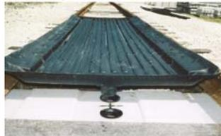
gauge pan should rest on the top of the ball of the rail, evenly on both sides.
