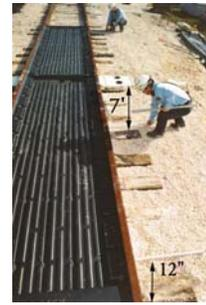
19. Install the “Bottom Field” pan by placing the downspout over the elastomeric gasket in the cross drain. With the flashing side of the pan resting on top of the rail, slide the outside wall of the pan over the field restraining clip.
