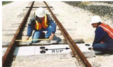
7. Install the cross drain with the raised rib 1" below the top of the cross tie on each side of the rail. This will allow proper drainage of the cross drain due to its unique built-in slope design. Check to make sure that the center of the cross drain is still centered with the center line of the track (tangent 28 1/4") and the cross drain is square to the rail.
