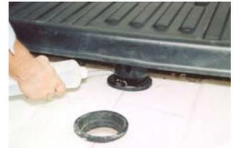
14. Insert the down spout in the rubber gasket by stepping on pan directly over the down spout as shown.
