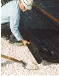
25. If there is the possibility that there will be a substantial amount of pedestrian traffic, it is recommended that a grated crosswalk be added to the pans for safety.
