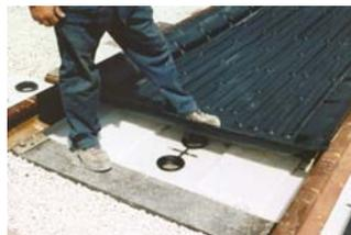
15. After the spout is installed in the cross drain, use the blunt end of a spike maul to force the lip of the pan under the ball of the rail. Carefully install the lip of the pan under the rail alternating from side to side working toward the end of the pan. Install all remaining bottom gauge pans by repeating previous steps.
