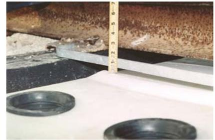
8. Place ballast around sides and ends of cross drain to hold it in place. Make sure that cross drain is kept square with the rail and the proper height maintained during the entire installation.
