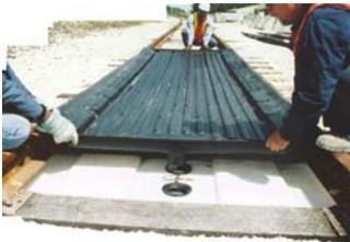
13. Lubricate the down spout and elastomeric gaskets with liquid soap to aid in the installation of the down spout into the cross drain.
