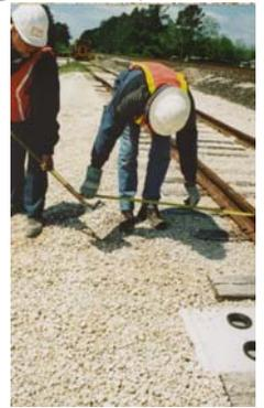
11. Once the cross drains, piping and ballast shoulders are installed, begin installing all the bottom gauge pans (see diagram). Each gauge pan will be marked either bottom or top. Field pans will be marked for B bottom and T for top. The field pans will be marked with a #1 or #2 to designate which side of the rail they will be installed.
