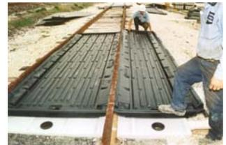
21. With the pan connected to the cross drain and the restraining clips holding the pan from sliding away from the rail, use the blunt end of a spike maul to carefully force the flashing edge under the rail.
