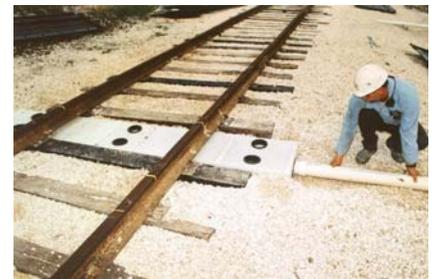
10. Ballast shoulders should extend 4'0" from the outside ball of rail on both sides of track (see diagram below). Ballast should be dressed off level with top of crosssties on the outside of the rail and 1/2" below the ties between the rails. The track structure is now ready to accept the HDPE Enviropans. The tops of the crosssties must be clear of all ballast stone.
