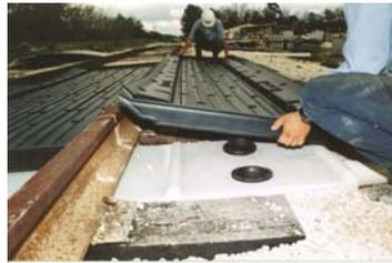
20. Next lubricate the downspout and elastomeric gasket with liquid soap. Insert the downspout into the opening with the elastomeric gasket in the cross drain by stepping on it.
