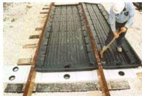
22. Install the #2 “Bottom Field” pans as shown in steps 15 through 18 on the opposite side of the rail from the #1 pan. After the bottom field pans are set, install the top field pans as depicted in steps 17 through 21. The top field pans will overlap the bottom field pans.
