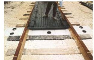
16. After all bottom gauge pans are installed, begin installing the top gauge pans as depicted in step 12. The top gauge pans will overlap the bottom gauge pans.
