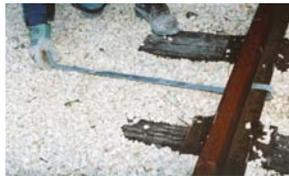
18. One clip should be placed midway of the pan and the second placed approximately one (1) foot from the end of the pan opposite the cross drain. (Use only two clips per field pan.)
